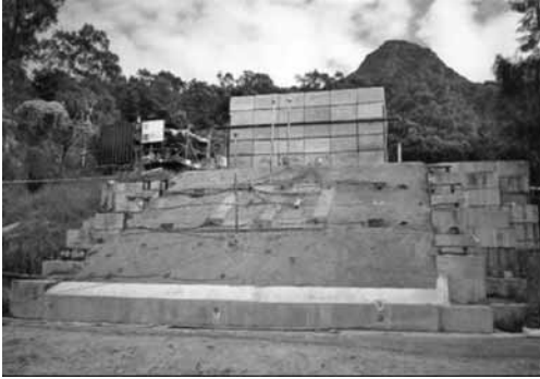
Figure 2. A view of the instrumented soil nailed slope site.
