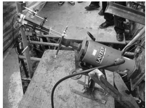
Figure 6. Field pullout test on soil nail with optical fiber strain sensors and electrical strain gauges.
